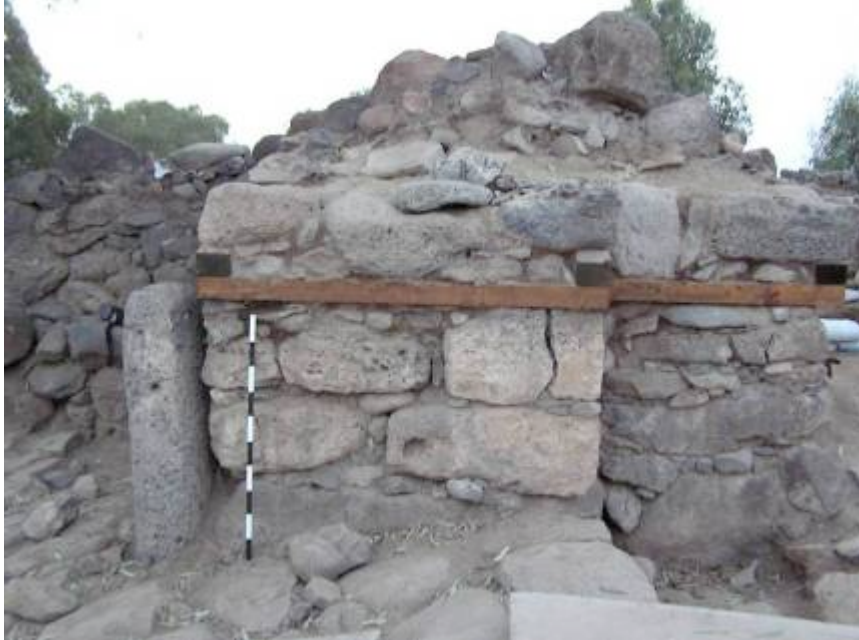
The southern door jamb at the inner gate, notice the wooden beams on top of three courses of stone.
